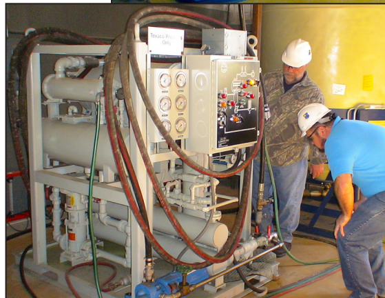
Stationary oil purifiers at the Oil Processing Facility
