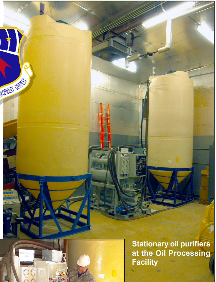
Personnel monitor oil purification system for pressure across the filter
