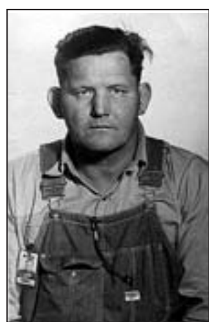
Tim's grandfather, John McNeese, can be seen here with his ARO (Arnold Research Organization) badge in 1957, when AEDC was still under construction. (Photo provided)
