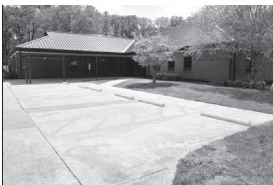
The newly remodeled Medical Aid Station parking lot was completed Wednesday. The sidewalk and walkway were repaired to comply with Americans with Disabilities Act guidelines and a new canopy was installed over the walkway. The slope of the old walkway was too steep, and there were cracks and unlevel ground. The new walkway provides a safer route to the front door, and the canopy allows for less rainwater to gather on the walkway and keeps inclement weather away from the doors, where elderly patients have more difficulty. The entire project took about five months. (Photo by Rick Goodfriend)
