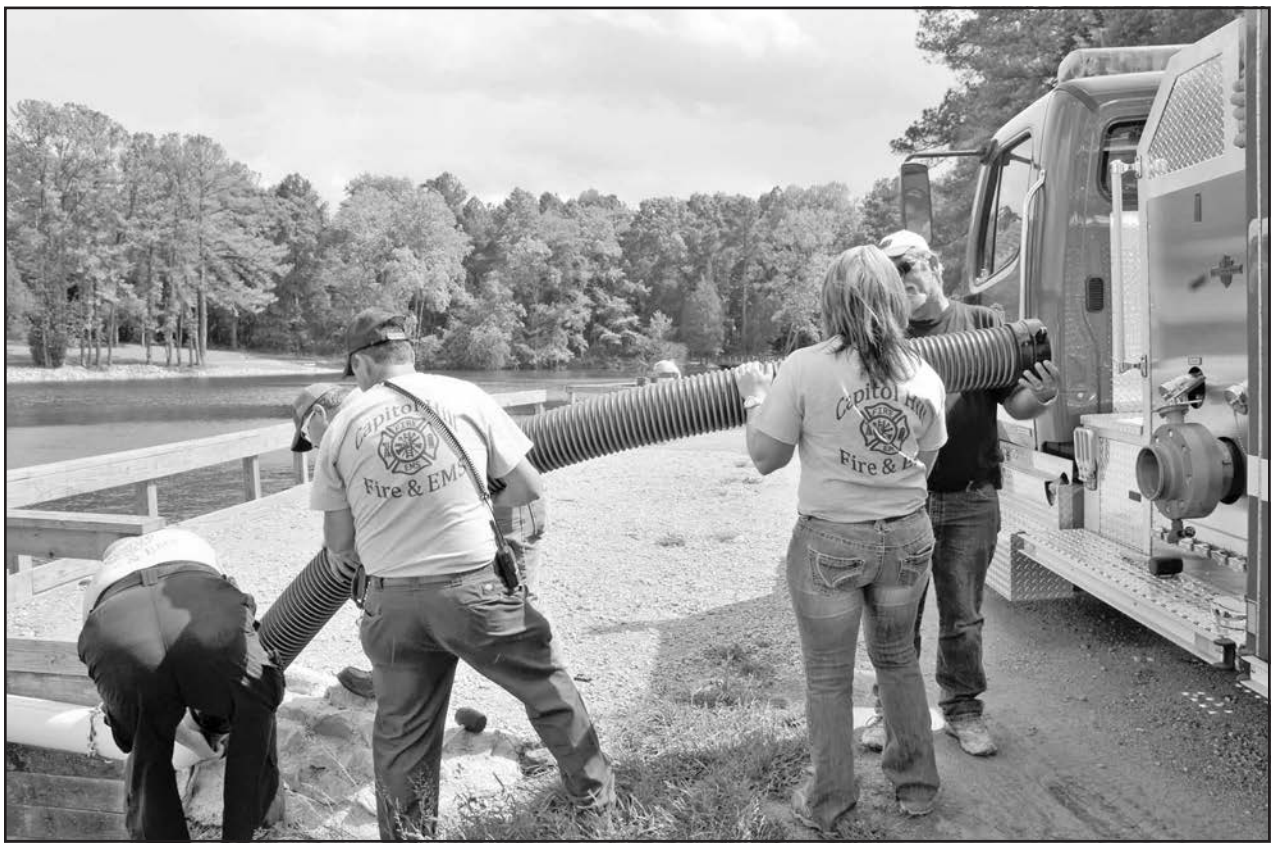
Members of the Capitol Hill and Arnold Air Force Base fire departments work together to perform a first draft of the dry hydrant installed at Morris Ferry Dock. Pictured in the first photo are Capitol Hill fire personnel hooking the fire truck up to the dry hydrant. As seen in the second photo, the fire hose successfully sprays water from the lake. Pictured in the last photo are AEDC fire personnel Odell Crutchfield (left) and Billy King (right) assisting in detaching equipment from the truck. (Photos by Jacqueline Cowan)
