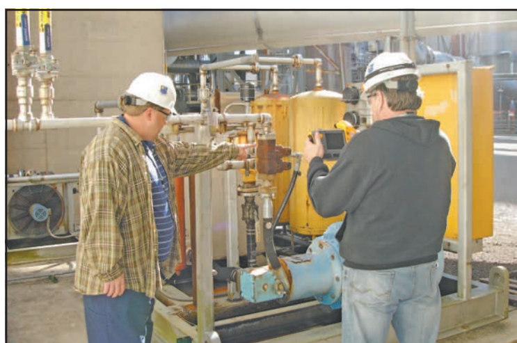
Dan Henley, infrared program lead (left), and Mike Rainey, Condition Based Maintenance outside machinist (right), take infrared temperature readings on a hydraulic unit in the Engine Test Facility A-Plant. This and other measures are taken as part of the Asset Health Assurance Program to ensure that equipment and infrastructure at AEDC are performing as needed. (AEDC photo)
